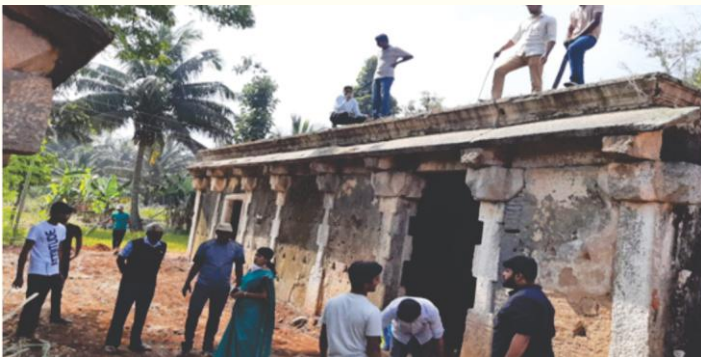
Restoration of an ancient Venkateshwara Temple at Srirangapatna
